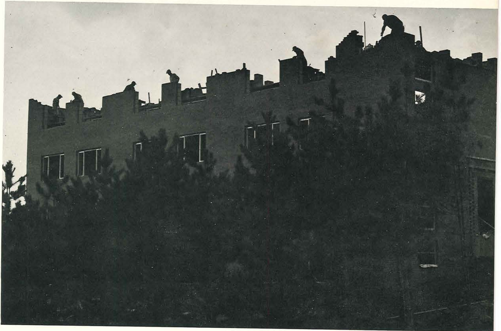
A new dormitory for sophomore men, in the process of construction . . .
