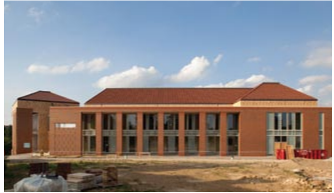
The South Elevation of Otto and Fran Walter Hall.
